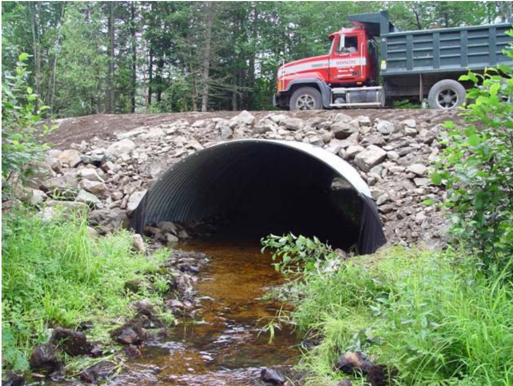
Figure 3-3: Examples of arch or bottomless culverts
