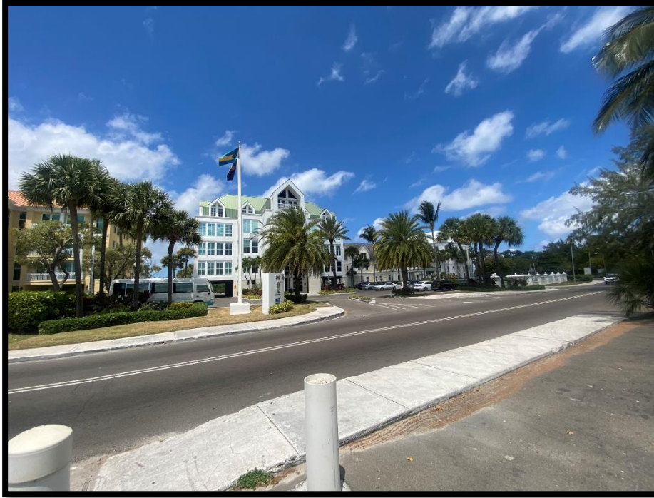
Figure 148. East Bay Street, access to the lift station and resorts located in front of Lift Station. Source: PlanEHS, 2024.
