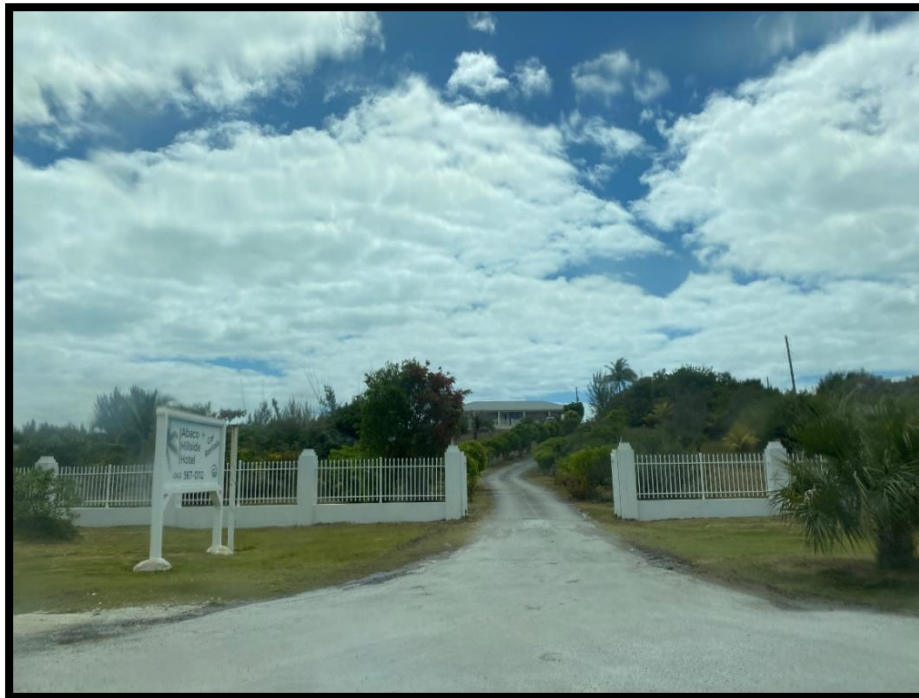
Figure 94. Abaco Hillside Hotel. Source: PlanEHS, 2024.
