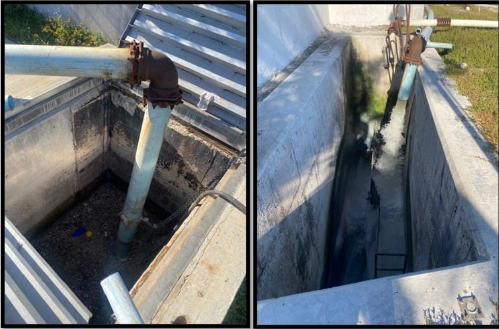
Figure 31. (a) 1 o well chamber and PVC bypass; (b) 2 o well chamber and PVC bypass. Source: PlanEHS 2024.
