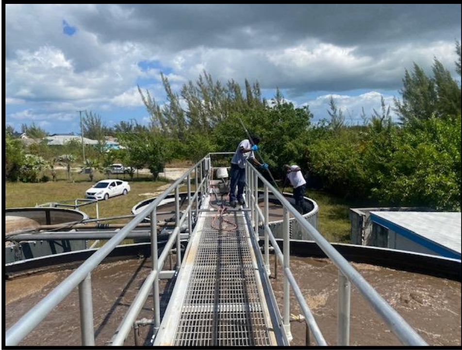
Figure 169. View of Aeration, Clarifier and Digestion Tanks. Source: PlanEHS, 2024.
