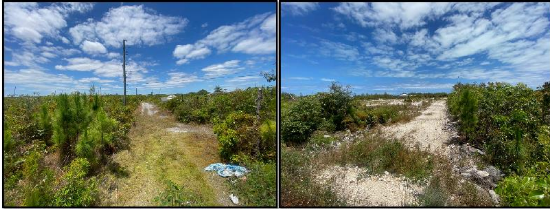
Figure 111. Uncleared and unpaved roads. Source: PlanEHS, 2024.
