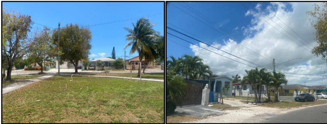
Figure 121. Surrounding houses to Flamingo C Lift Station on Bahamas Boulevard. Source: PlanEHS, 2024.
