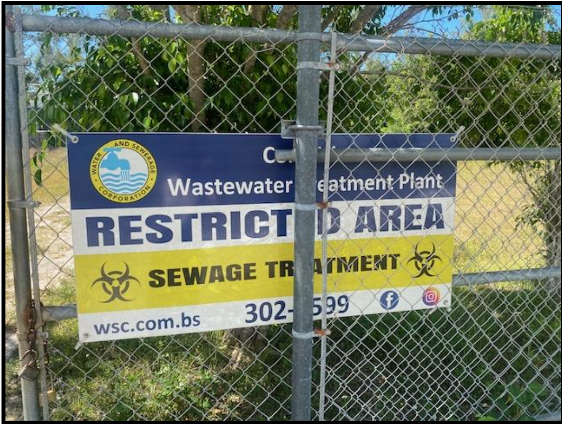
Figure 167. Gated fence entering Coral Vista Wastewater Treatment Plant. Source: PlanEHS, 2024.
