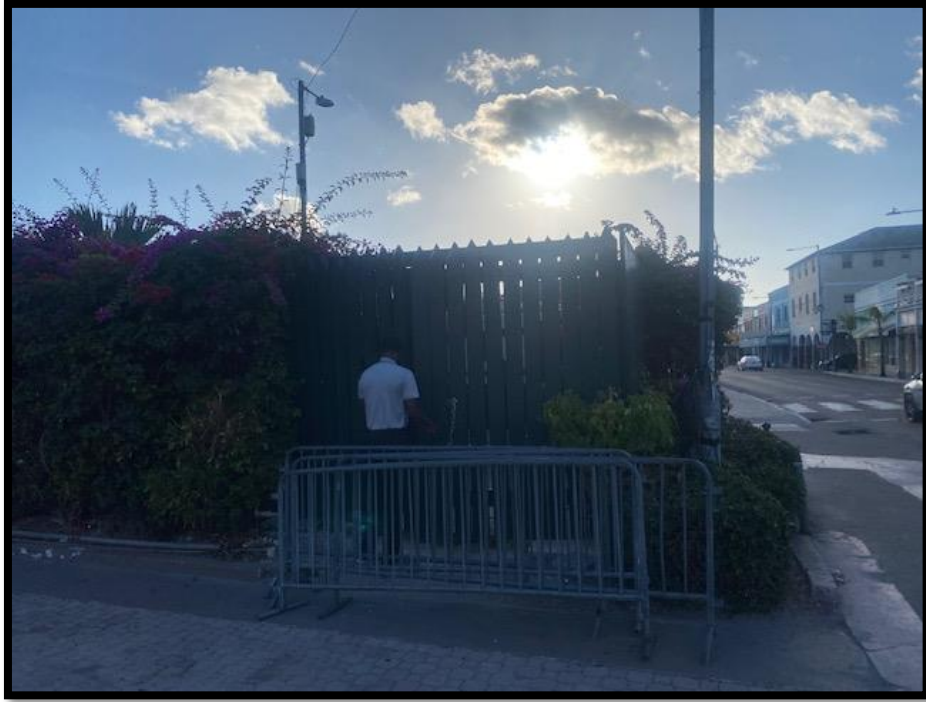
Figure 23. Rawson Square Lift Station. Source: PlanEHS 2024.
