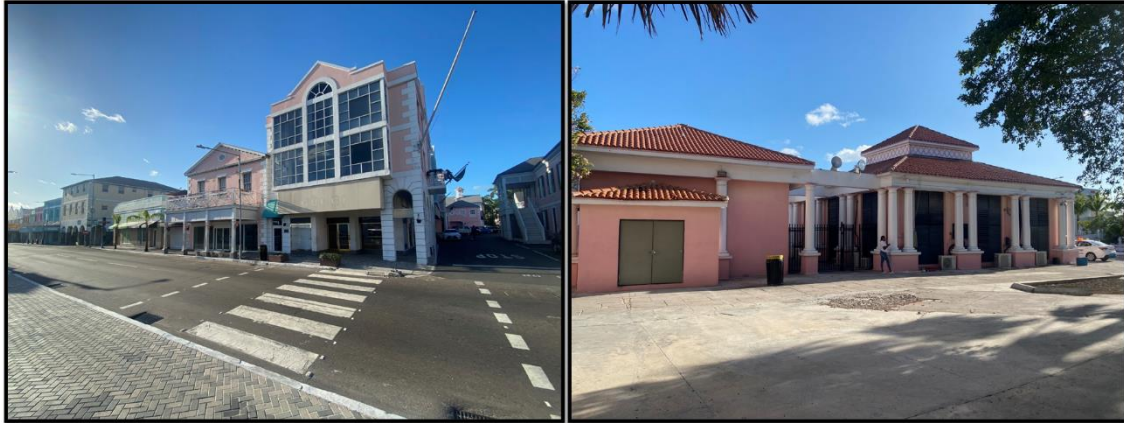
Figure 136. Surrounding buildings from Rawson Square Lift Station. Source: PlanEHS, 2024.
