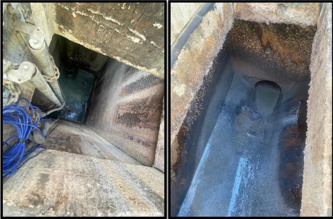
Figure 27. Well chamber and secondary chamber. Source: PlanEHS, 2024.
