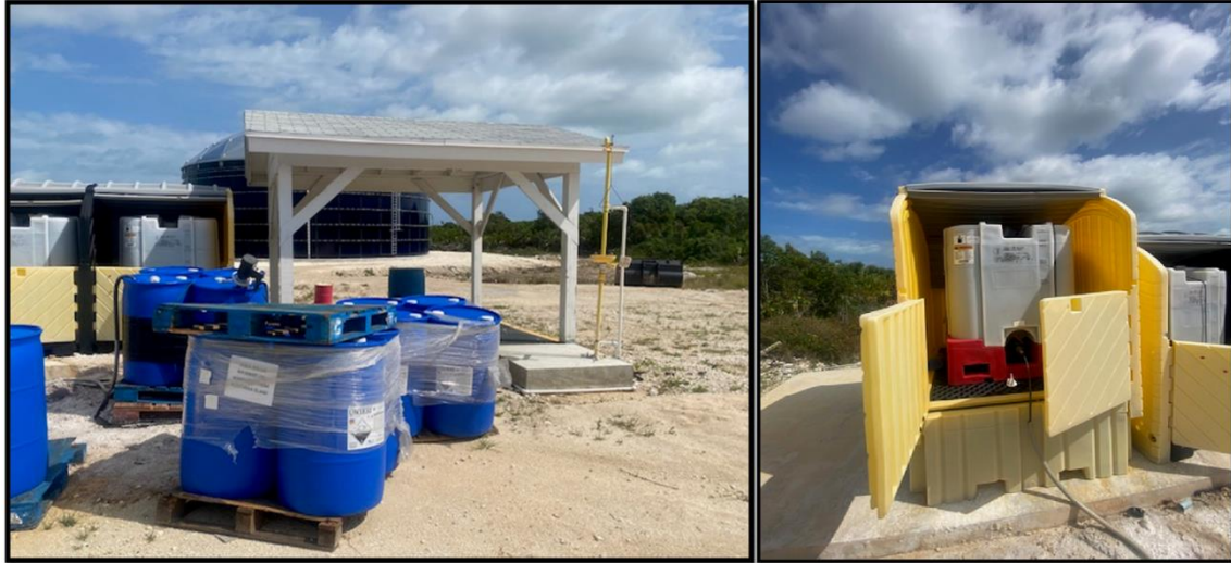
Figure 154. Sulfuric Acid Solution to treat feed water. Source: PlanEHS, 2024.
