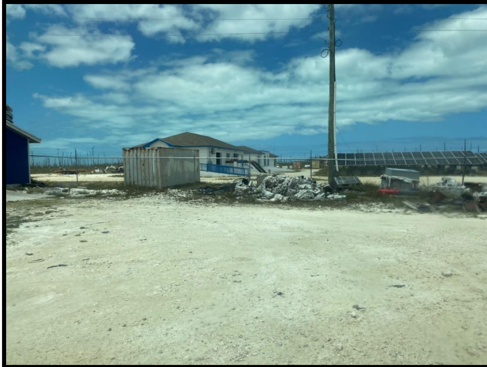
Figure 160. Pumping Station, Storage Building, Generator Building and Solar Plant. Source: PlanEHS, 2024.
