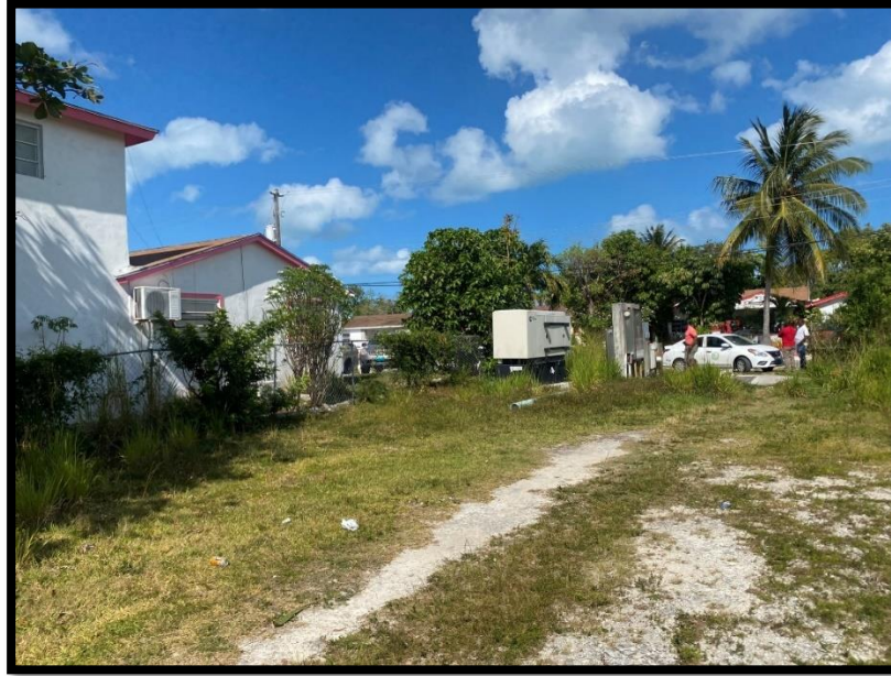
Figure 128. Adjacent residential home of Elizabeth East Lift Station view from unpaved path that leads to Trinidad Way. Source: PlanEHS, 2024.
