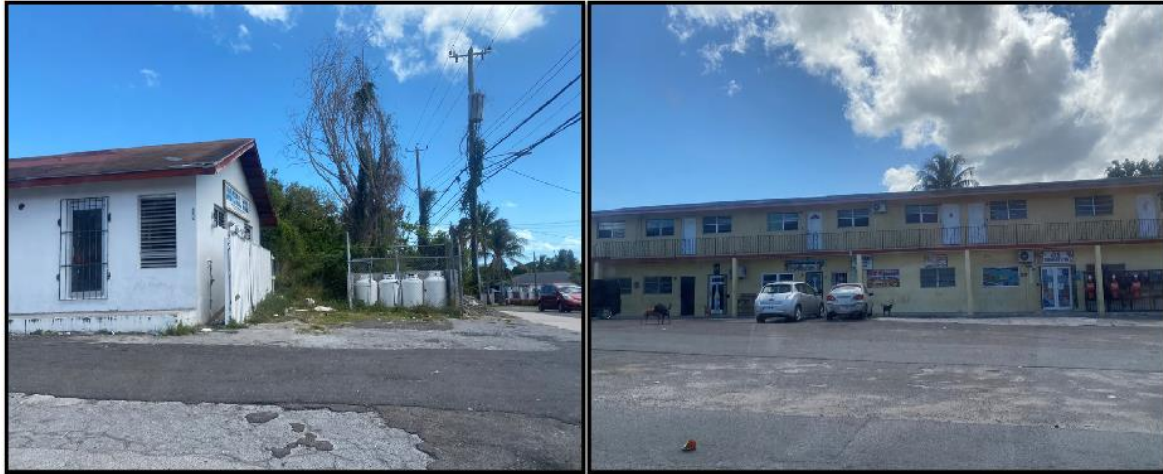
Figure 89. Businesses in Nassau Village: (a) Car Wash; (b) Convenience store. Source: Plan EHS, 2024.
