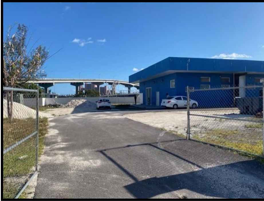
Figure 29. Entrance to Malcom Park Lift Station and nonoperational plant (blue building). Source: PlanEHS, 2024.
