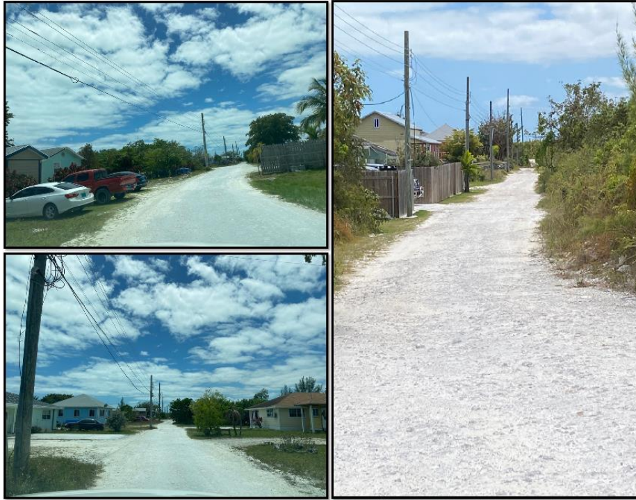
Figure 107. Overhead electricity poles in Sweetings Tract. Source: PlanEHS, 2024.
