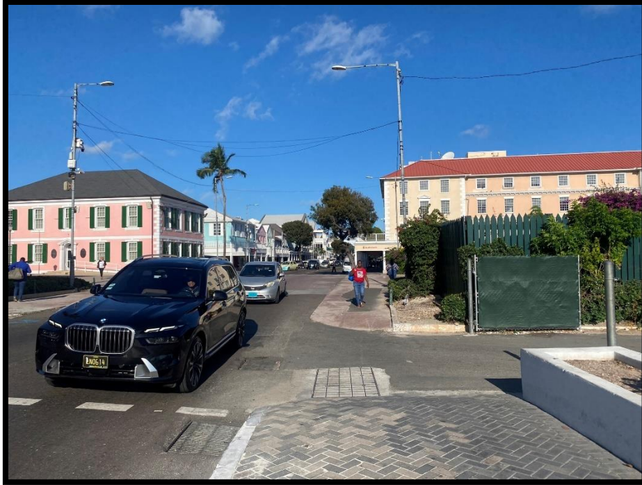
Figure 133. Bay Street with overhead lighting and sewer system and view of Rawson Square Lift Station (green fenced). Source: PlanEHS, 2024.
