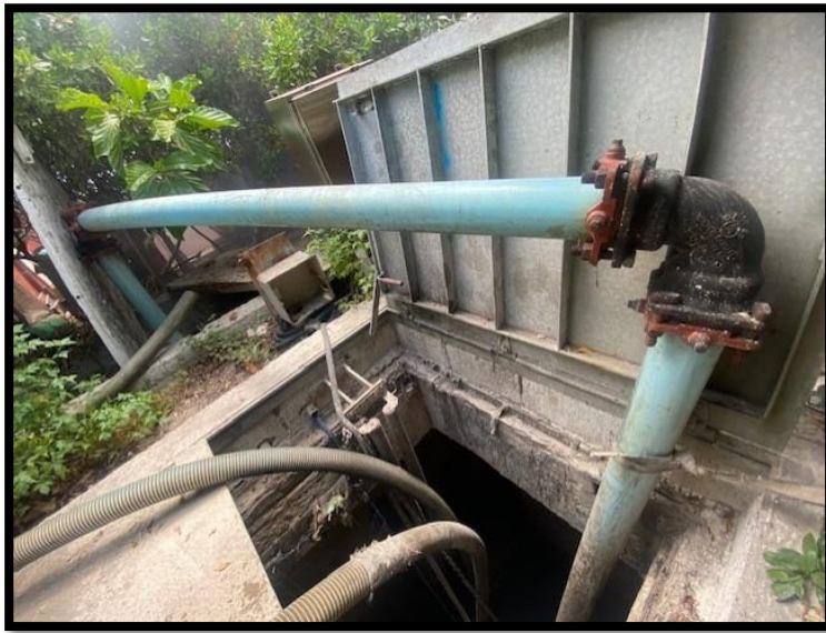
Figure 150. Temporary bypass needed for operation. Source: PlanEHS, 2024.
