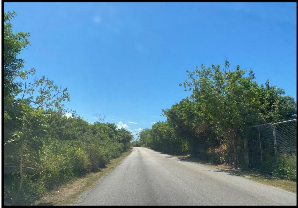
Figure 74. Miller Road mains extension. Source: Plan EHS, 2024.
