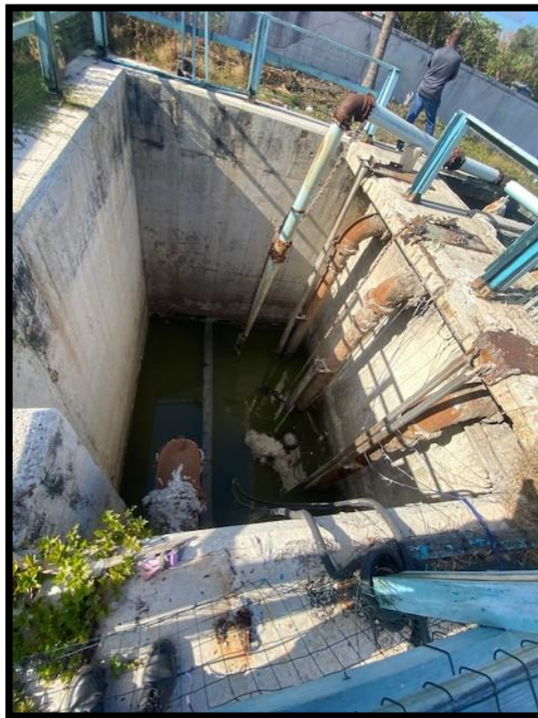
Figure 32. 3 o well chamber and bypass from blue building. Source: PlanEHS, 2024
