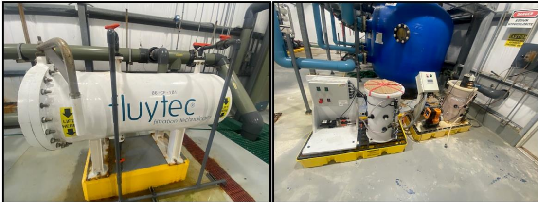
Figure 155. Potabilization Process: (a) Filtration prior to RO membranes; (b) Chlorination after RO process. Source: PlanEHS, 2024.
