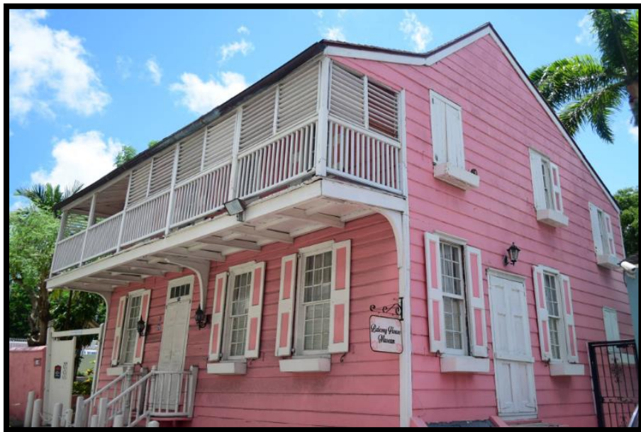
Figure 70 – Balcony House near a proposed project site (Rawson Square). Source: AMMC website
