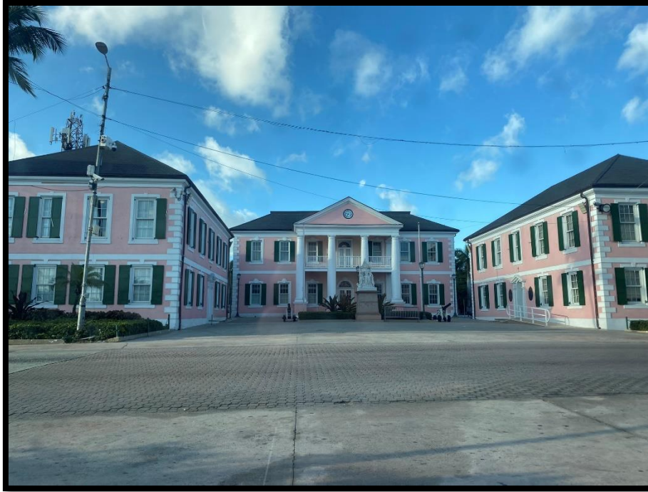
Figure 134. Parliament Square in front of Rawson Square Lift Station. Source: PlanEHS, 2024.
