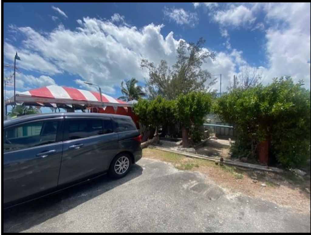
Figure 35. Location of Montague Lift Station, adjacent to local vendor. Source: PlanEHS, 2024.
