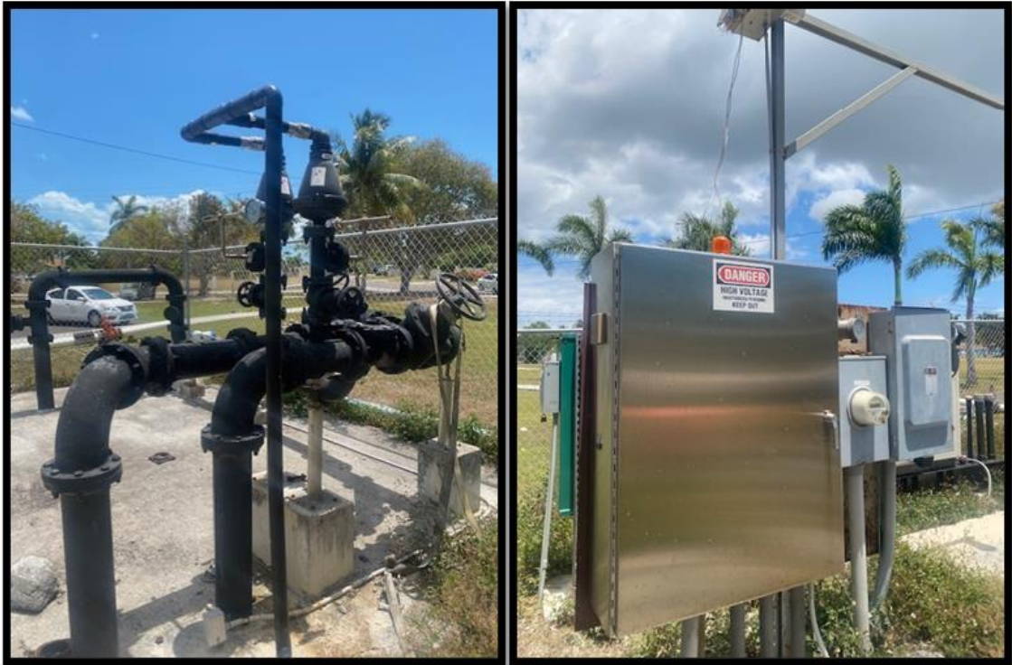
Figure 15. (a) Overground valves; (b) Pump Control Panel. Source: PlanEHS, 2024.
