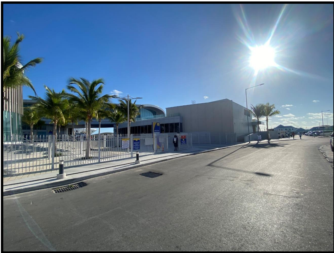
Figure 137. Bahamas Cruise Terminal, 130 ft from Rawson Square Lift Station. PlanEHS, 2024.
